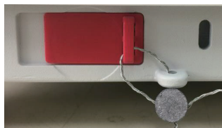
Locked with Wire Seal
