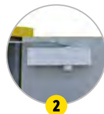
2 Self-closing door with thermo-fuse
