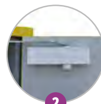
2 Self-closing doors with thermo-fuse
